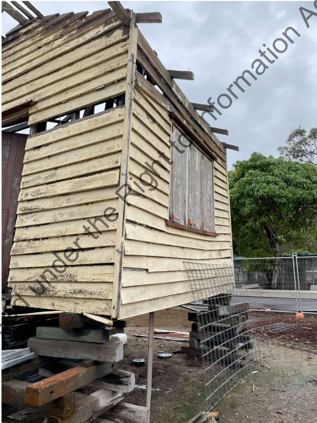
Figure 14 – Collapsed roof framing
