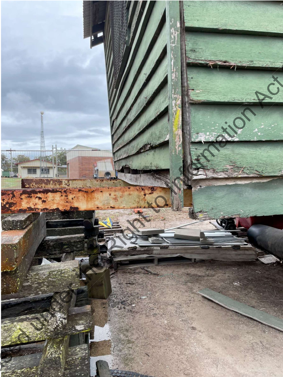
Figure 8 – Existing bearer distorted.
