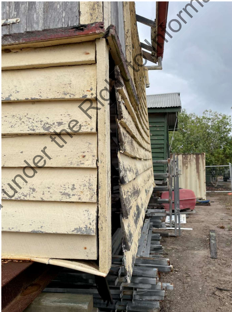
Figure 10 – Example of failure of fixings
