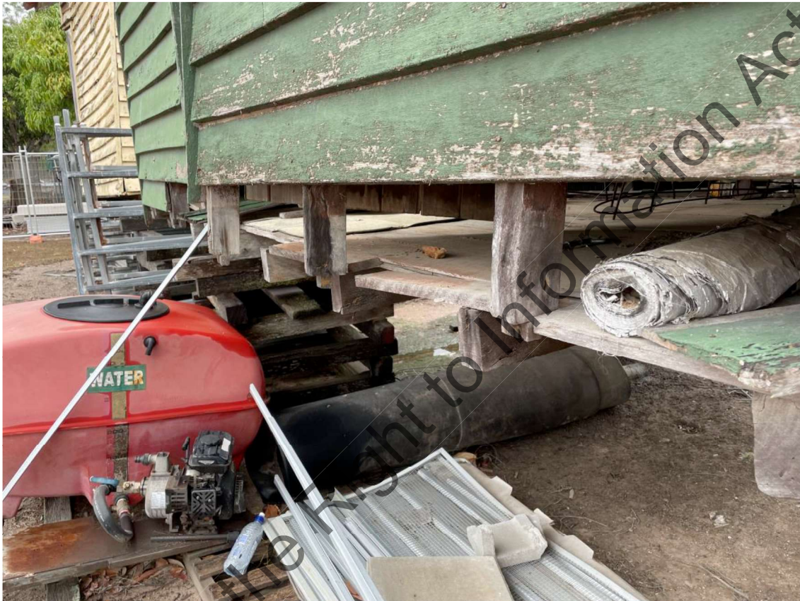
Figure 9 – Existing bearer missing.
