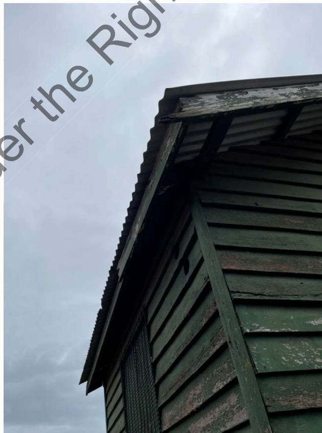
Figure 13 – Example of decay in roof framing.
