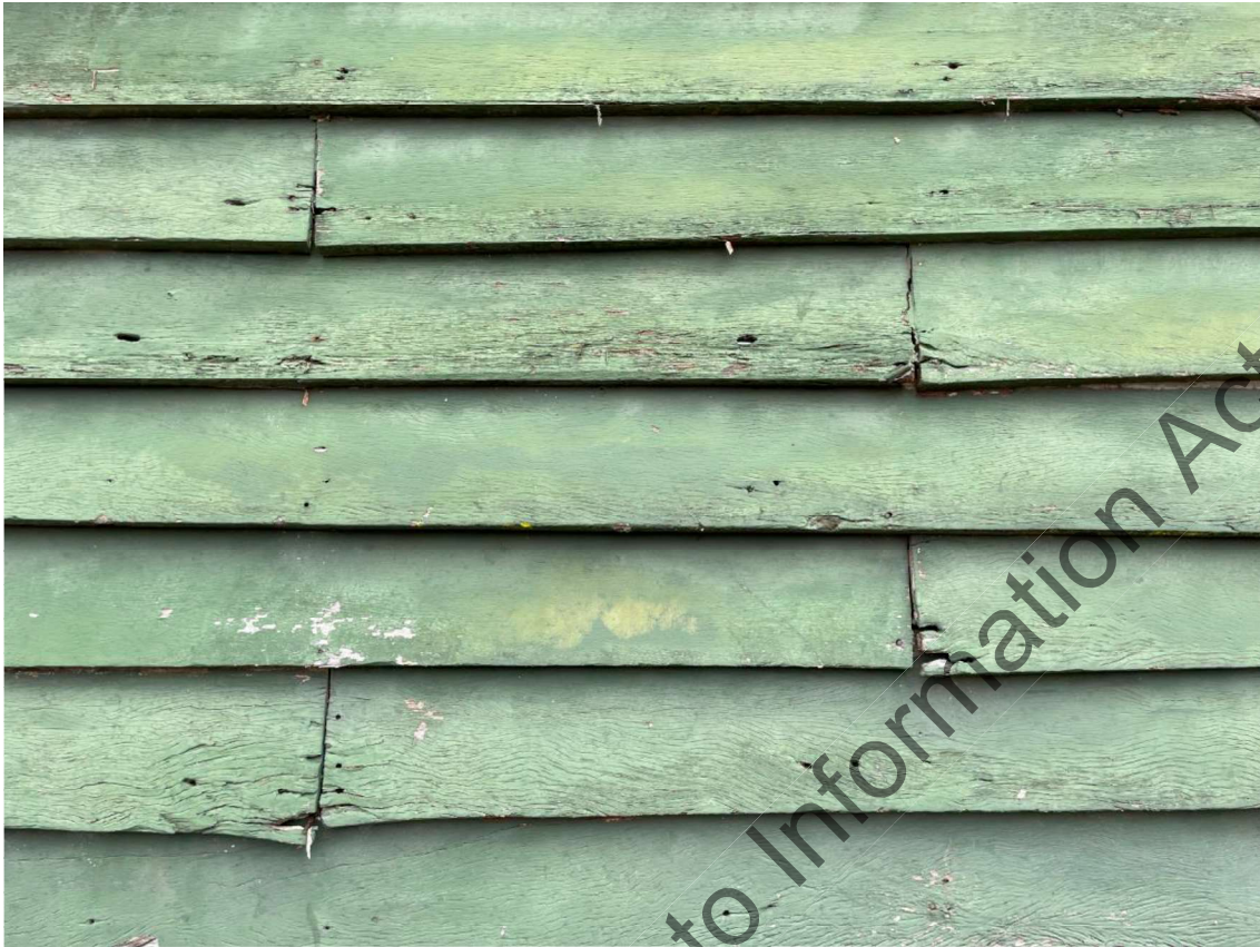
Figure 12 – Example of dry rot in cladding.
