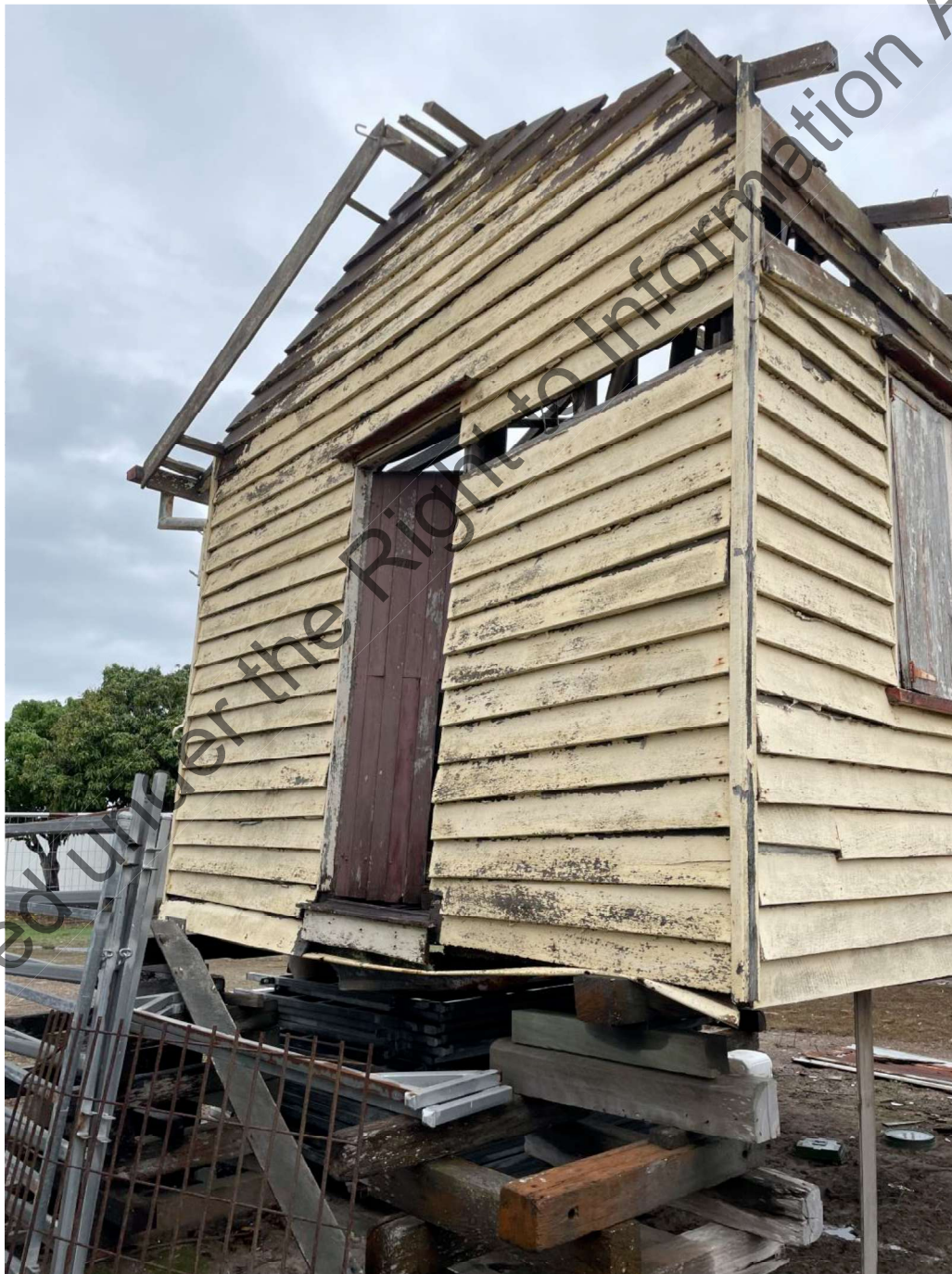
Figure 7 – Existing wall frame distorted.
