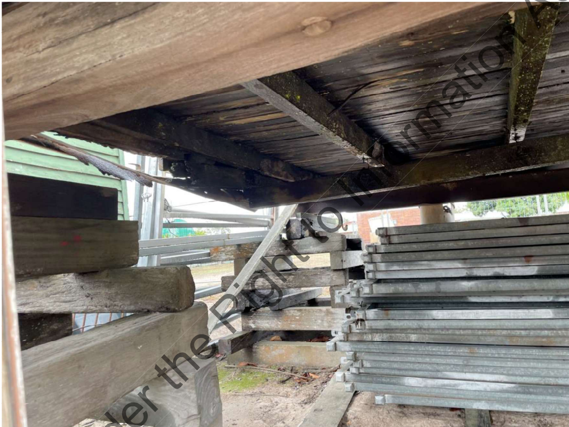
Figure 15 – Partial collapse to floor framing.
