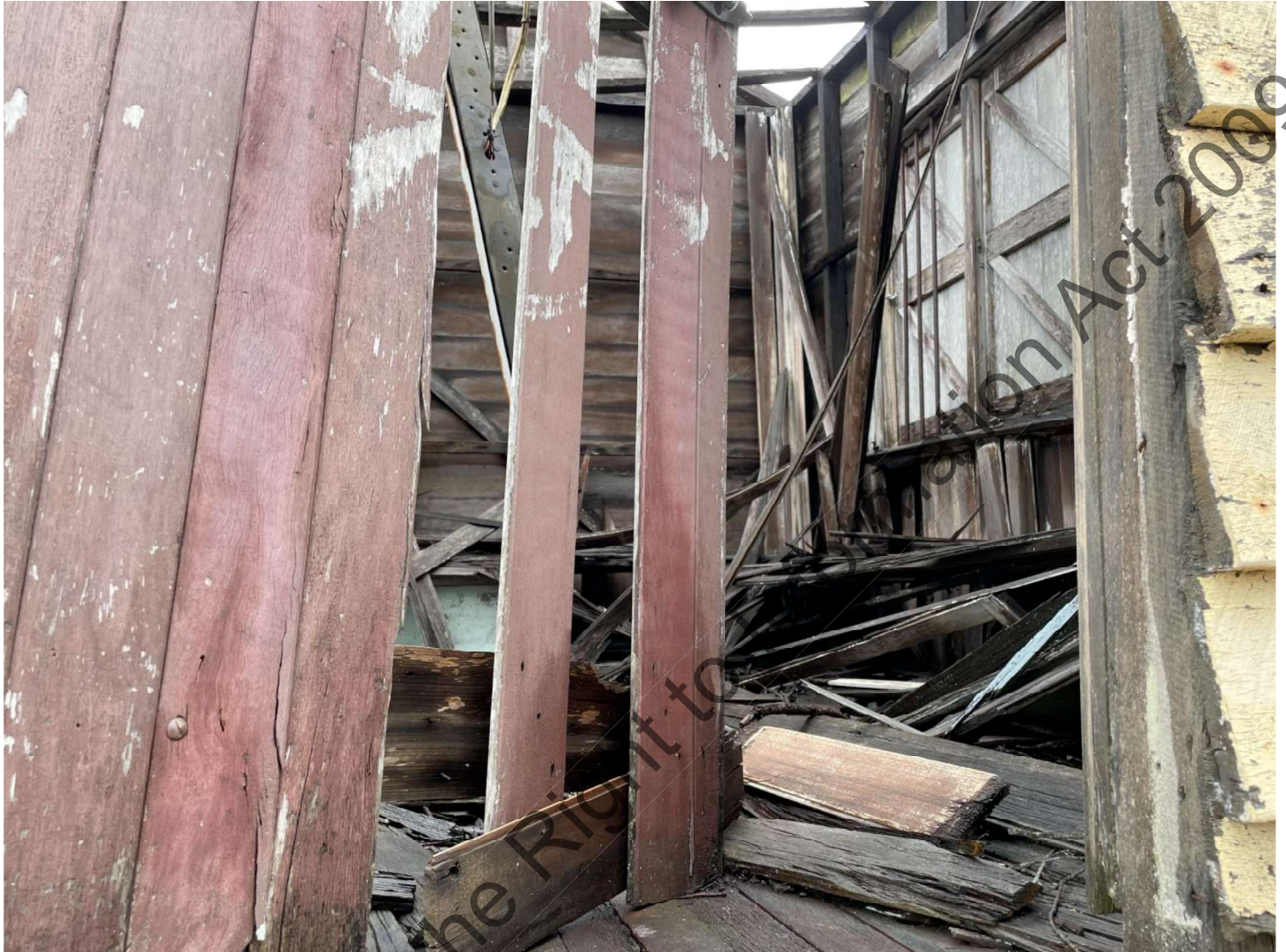
Figure 14 – Collapsed roof framing inside the hut
