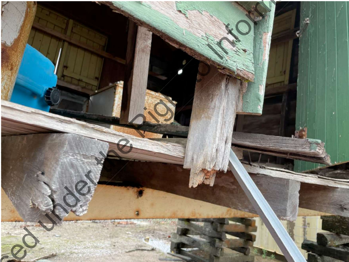
Figure 11 – Example of signs of termites
