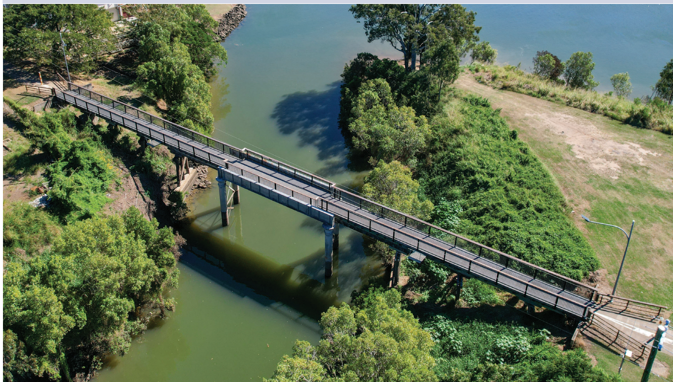
Saltwater Creek foot bridge, Bundaberg East.
