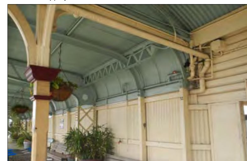
Detail of western platform extension illustrating change in building style and material.
