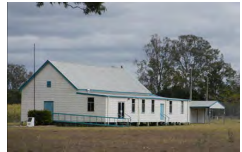
View to front and eastern elevation.
