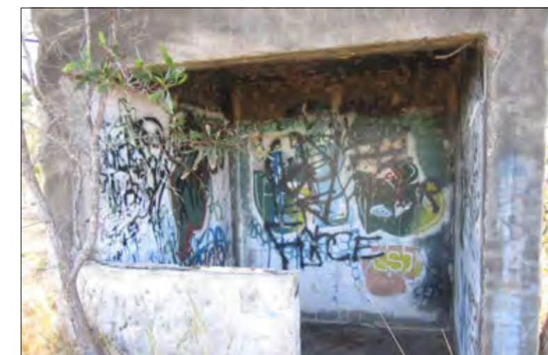
Close-up of door entrance and observation window.
