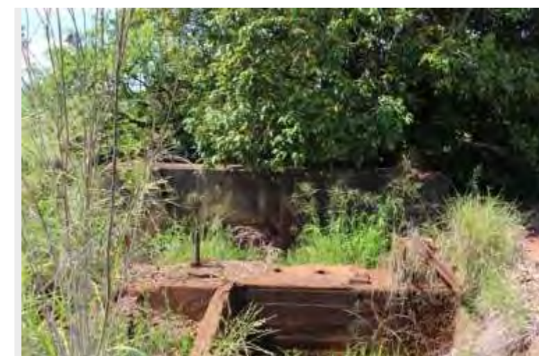
Footings of crushing plant.
