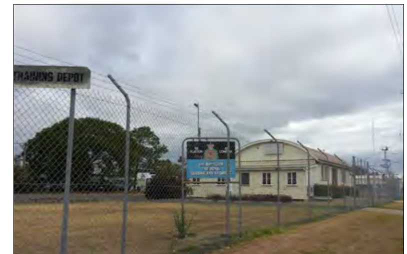
View of drill hall and setting from Quay Street.
