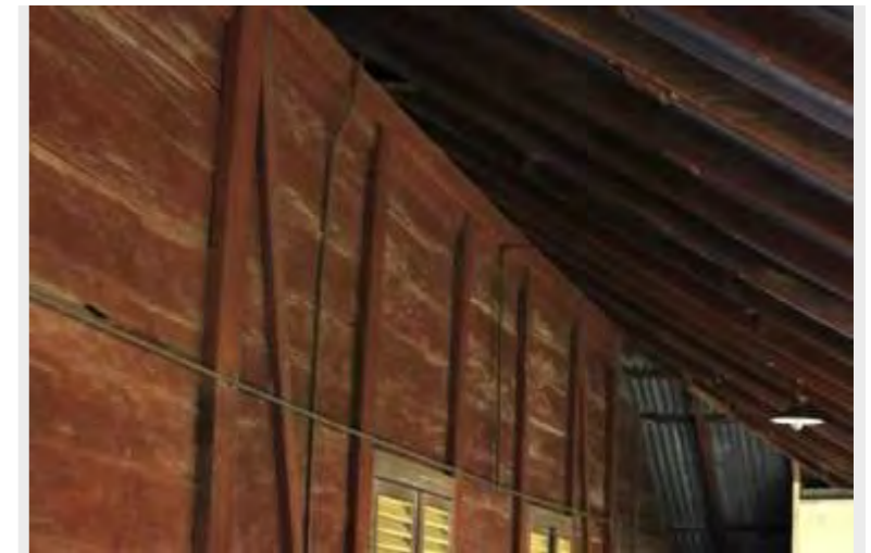
Detail of slab construction.
