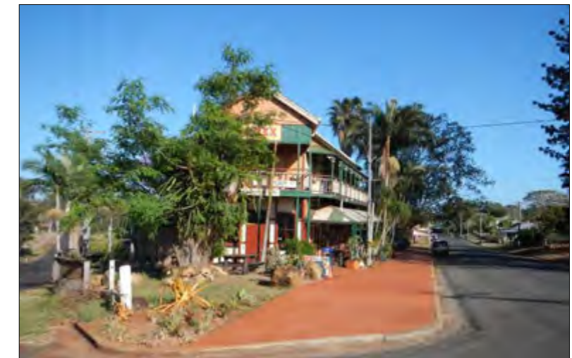
View to corner entrance.
