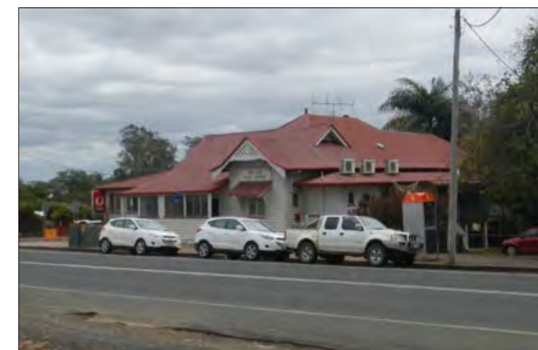
View to front and eastern elevation.
