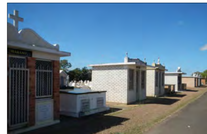
Mausoleums and vaults section.
