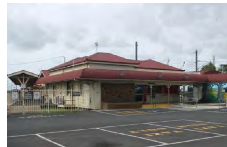
View to entrance from carpark.
