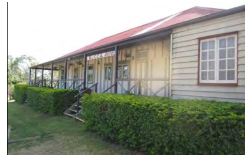
Entrance to Bucca Hotel, view to southwest.
