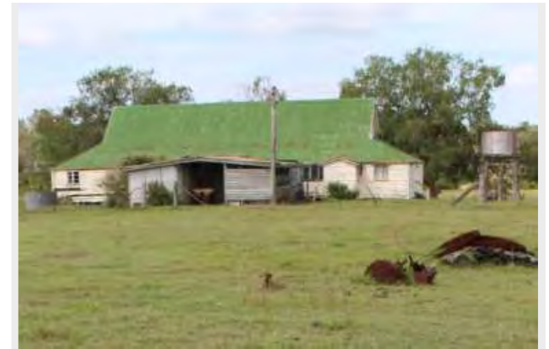
View to south-western elevation.
