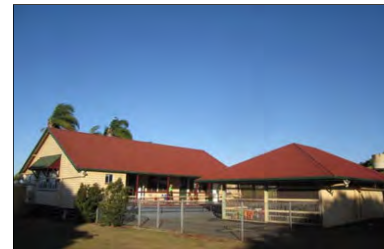
School and shelter building, view to south.
