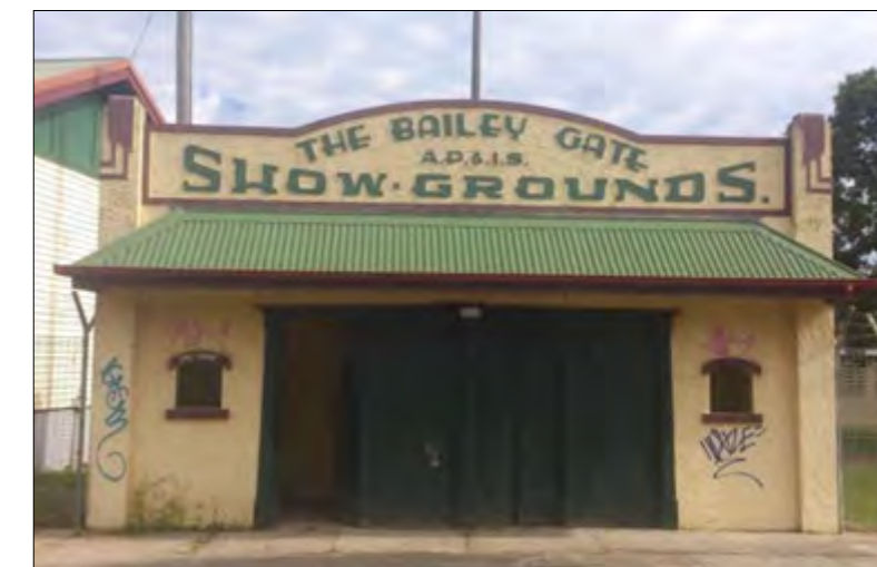
Front entrance facing Burrum Street, view to southwest.
