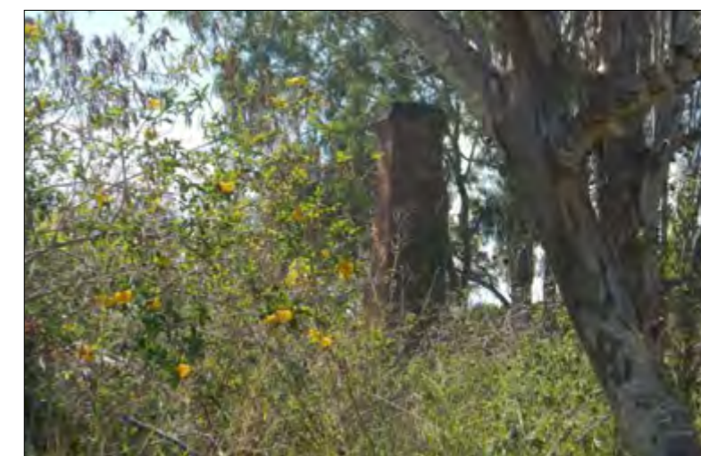
Brick chimney in the south-western section.
