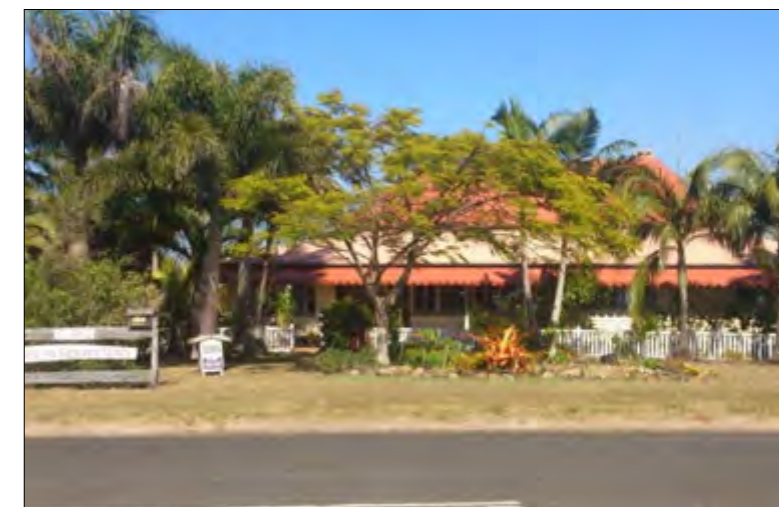
Front elevation, view to west.
