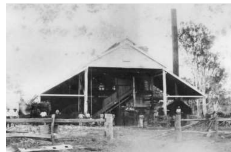
John Oxley Library, File#2395885. Caption: 'Crushing mill, Pemberton Grange sugar plantation, Bundaberg district, 1898'.
