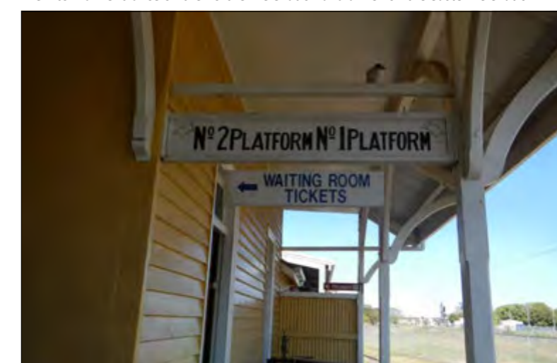
Close-up of platform awning.
