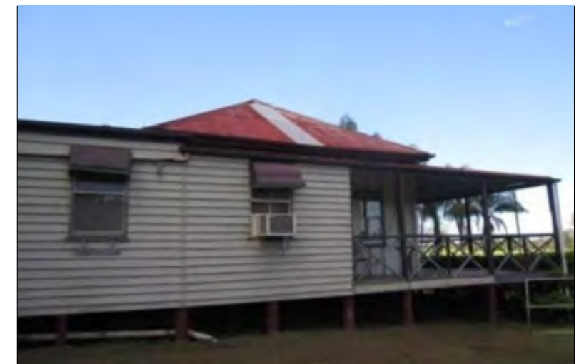
View to southern elevation.
