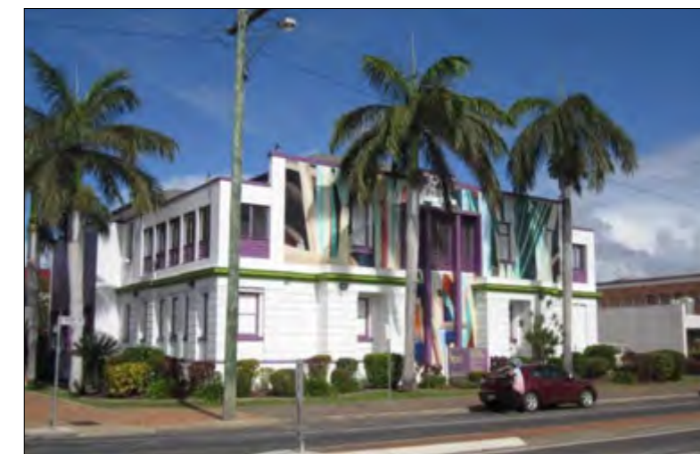
View to front and east elevation from Quay Street.
