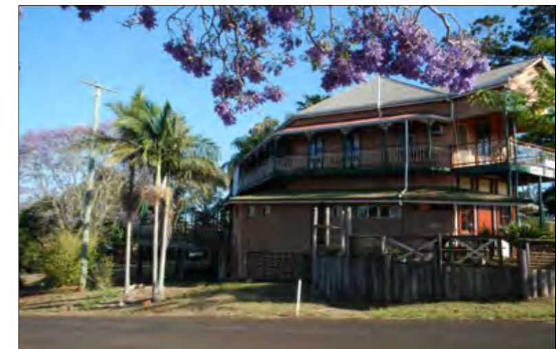
View to southern elevation.
