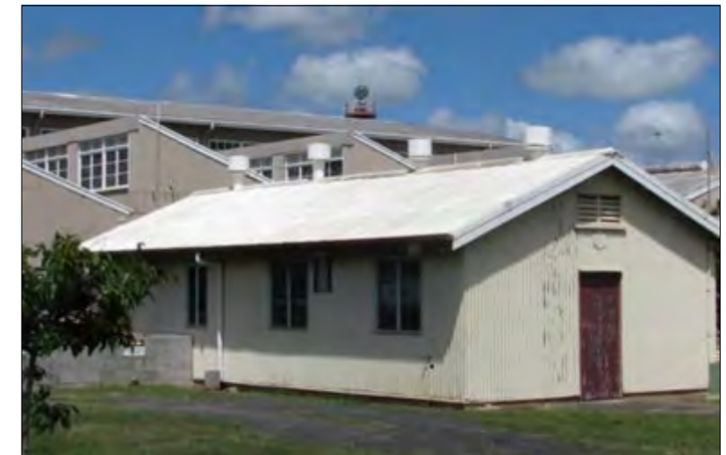
Former inflammables store.
