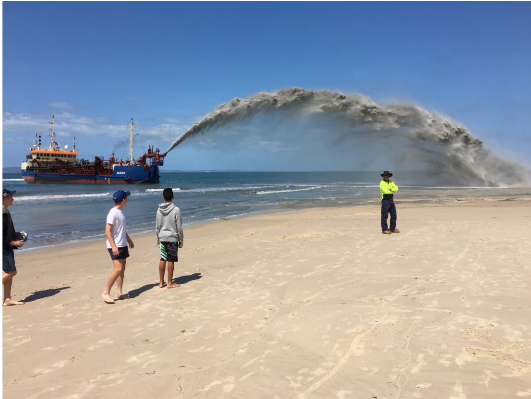
FIGURE 5-1 BEACH NOURISHMENT – OFFSHORE SAND PUMPING
