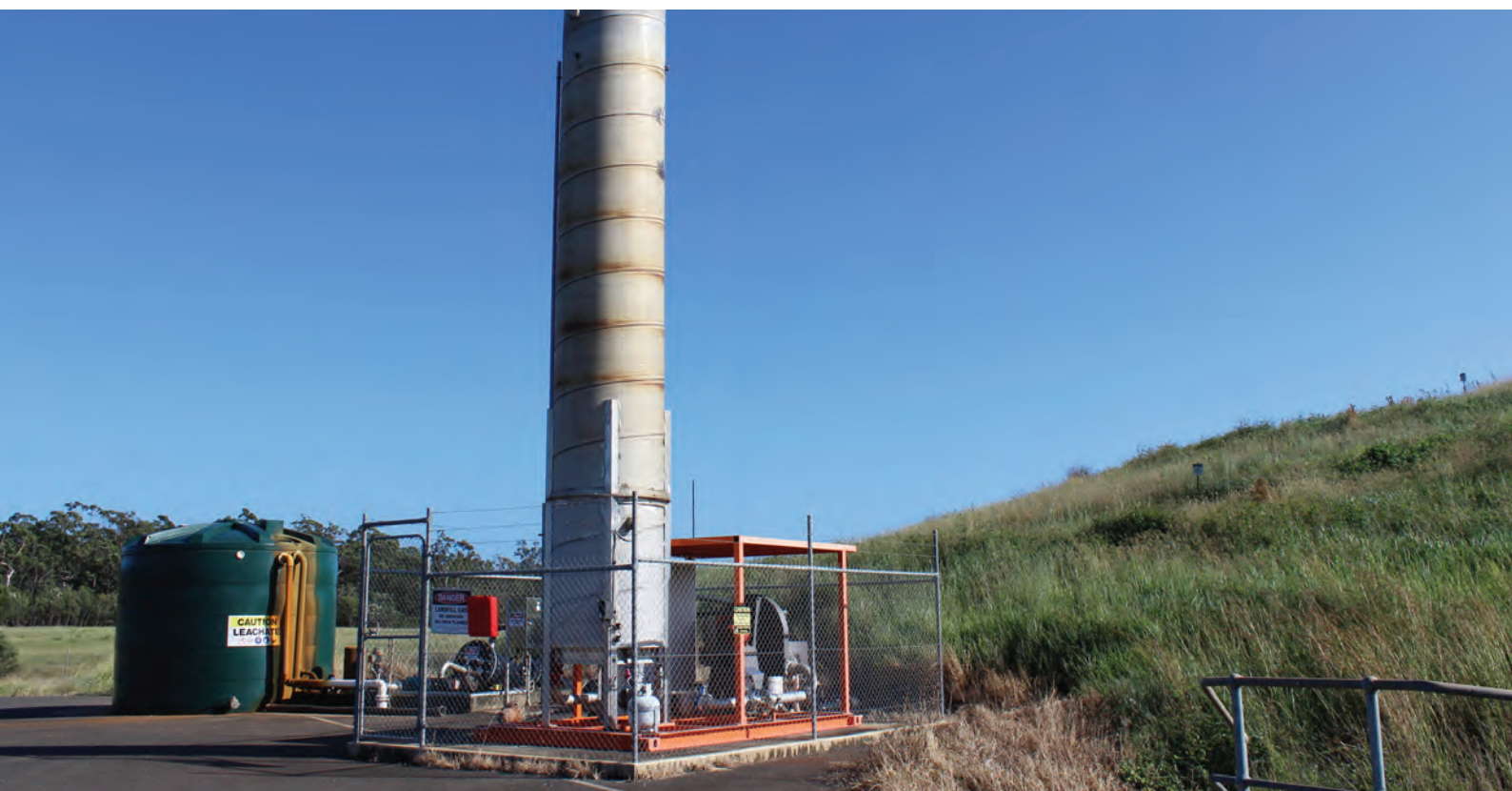
Landfill flaring system at the Cedars Road waste facility
